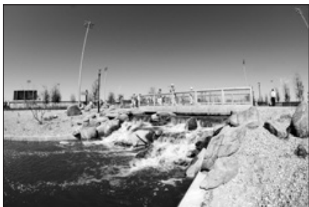
A bridge and waterfall greet fans on approach to the park.
